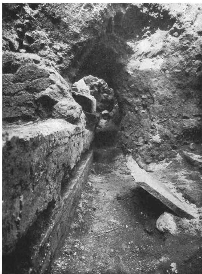
Fig. 111 — S. Lorenzo f.l.m. Basilica maior , dig 5, foundation wall of colonnade, from west (Photo: Sansaini).
